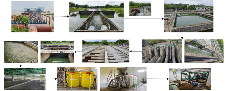
Fig. 2. Photos of stages of water treatment by RWASA
